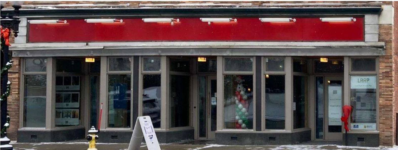
The former F.W. Woolworth sign band and granite bulkhead at 19 Park Street was retained, restored and the storefront made ADA accessible.
