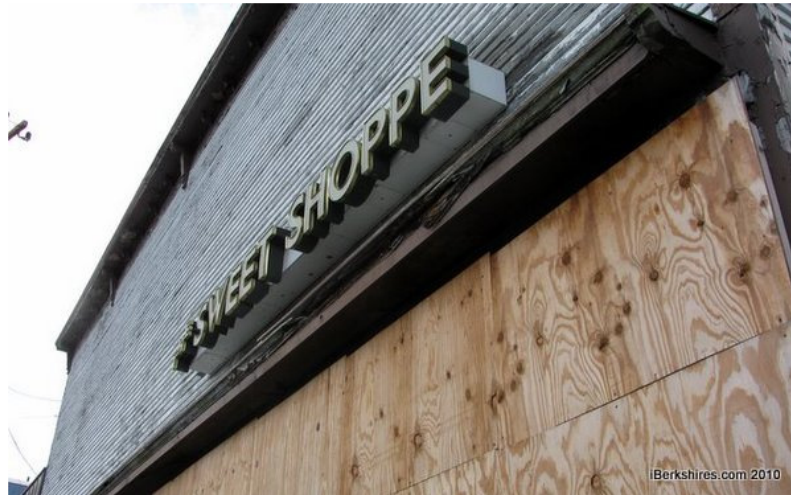
The Sweet Shoppe was demolished on Wednesday.
