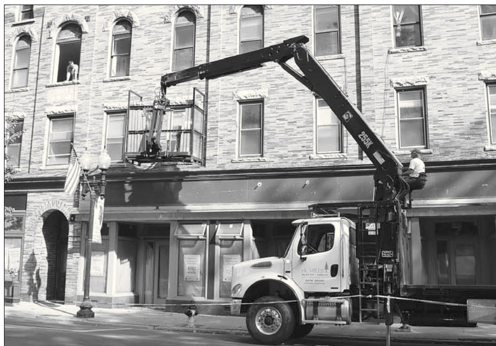
In early October, building materials supplier R.K. Miles delivers a shipment of new windows that will be installed in the upper floor of the Mausert Block as part of the mixed-use redevelopment project.
